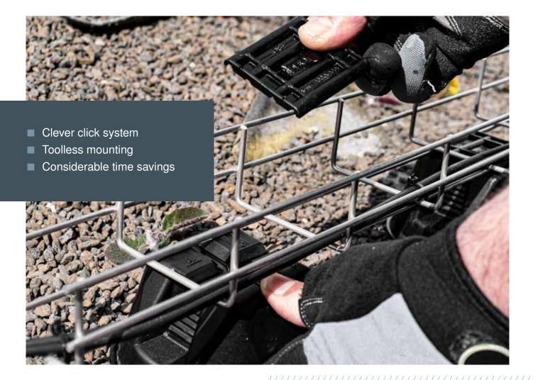
Provides the decisive installation benefits for the mounting of GR-Magic<sup>®</sup> mesh cable trays on flat roofs quickly and simply: the plug-in mesh cable tray adapter for the 165 MBG roof conductor holder.
